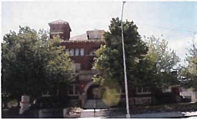
Human Resources presently occupies the Romanesque style Georgia Hall, a portion of Grady Hospital's original building. Photo by Joy Melton
