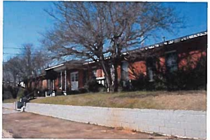
The Americus Colored Hospital was one of the few healthcare facilities in Georgia where African American doctors, nurses and pharmacists could practice in the early 20th century. A Georgia Historical Society marker was dedicated on the hospital grounds on January 24, 2009.
