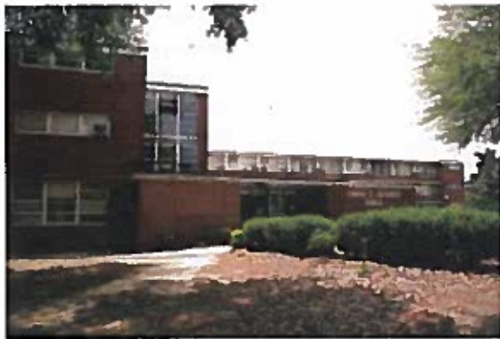
The current Jeanes Hall was constructed in 1952. It is an International Style building that forms the second historic core of the campus. Currently used as a men's dormitory, the Campus Historic Preservation Plan identified this building as eligible for listing in the National Register of Historic Places.
