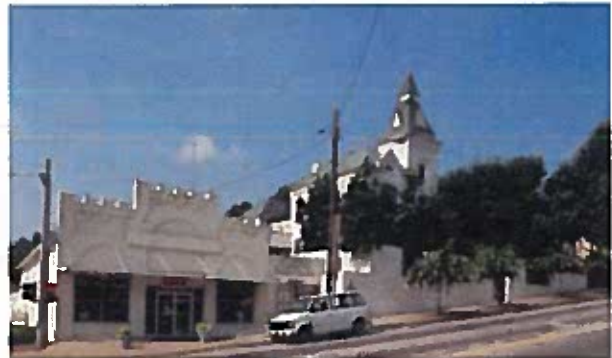
Today, the former Troup County Jail houses the Chattahoochee Valley Art Museum in the LaGrange Commercial Historic District.
