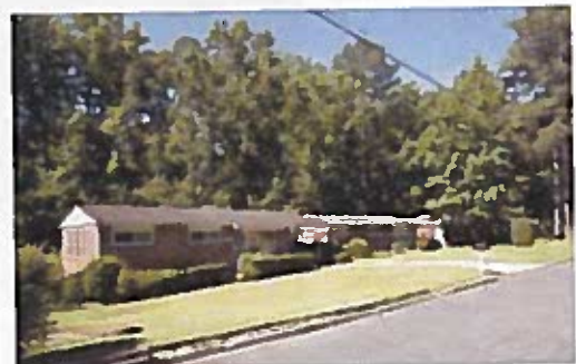
These "compact" Ranch Houses were constructed with brick veneer, the most popular building material in Georgia.
