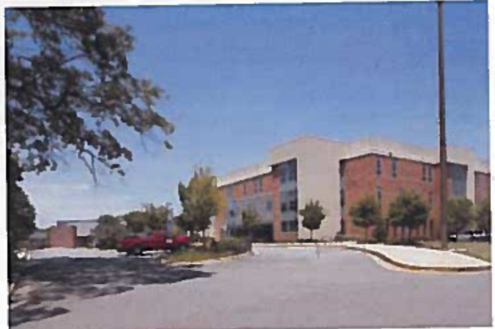
Frederick Douglass High School opened in the fall of 1968 in the southeast periphery of Collier Heights. The school features the Brutalism style of architecture that is monolithic in massing and features minimum windows. The 2004 auditorium and gymnasium (on the left) were not contributing resources in the Collier Heights nomination. Photo by James R. Lockhart
