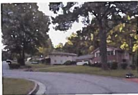
Split-Level houses are common in this subdivision. Photo by James R. Lockhart
