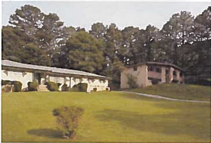
The Ranch house on the left uses metal shutters for ornamentation. The house on the right is a Split-Foyer. Its distinctive characteristics are an entrance at grade level with the main living area on the upper level while the lower level provides ample space for a recreation area.
