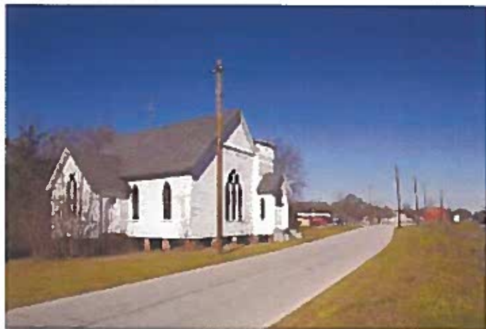
Haven Memorial Methodist Episcopal Church was constructed from 1888-1891. The church building sits on raised piers and is a wood structure with Gothic-Revival design features and stained glass windows.
