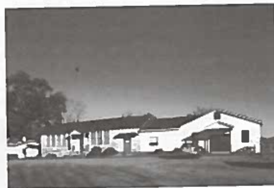
A wood building was constructed on the campus as enrollment increased. Its design was influenced by the Community School Plans . Photo by James R. Lockhart
