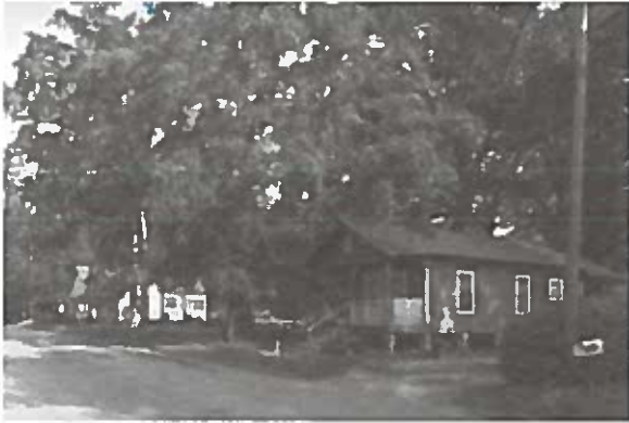
These are examples of a bungalow (left) and a shotgun house (right) on Festus Street in the Dewey City Historic District.
