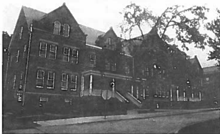
Morehouse-James Hall (1901) has consistently been used as a dormitory. It was renovated in the 1970s to provide housing for 85 students.
