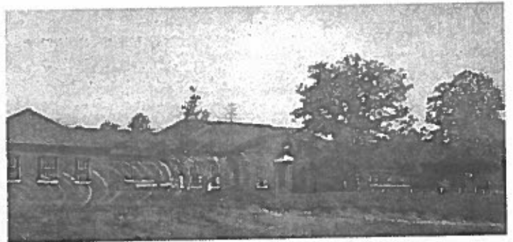
This historic photo of the dormitory on the Gordon Campus was taken shortly after its construction in 1939.
