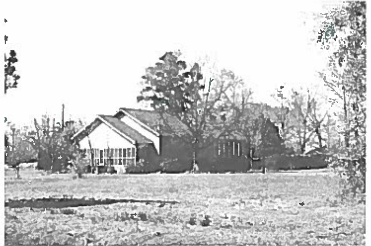
The Omaha Rosenwald School in Stewart County is the first school identified in the inventory that was converted to a residence. Photo by Jeanne Cyriaque
