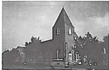
The 1801 St. John wooden building was listed in the National Register of Historic Places on June 17, 1982. The 1897 brick building was listed in the National Register of Historic Places on July 5, 1990.
