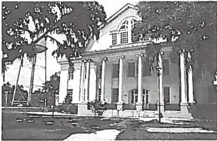
Hill Hall was completed in 1901 by students who were supervised by by trade instructors. The building materials consisted of masonry, wood and metal, and the students received proficiency certificates in the mechanical arts program that was offered at the college. Photo by Jeanne Cyriaque
