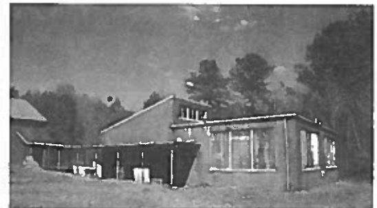
A walkway was added in the 1950s to connect the school to restrooms and a cafeteria. Photo by Jeanne Cyriaque
