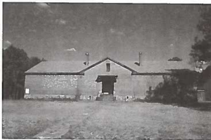
The windows and front entrance of the Eleanor Roosevelt School were covered with brick to prevent vandalism. Photo by Jeanne Cyriaque
