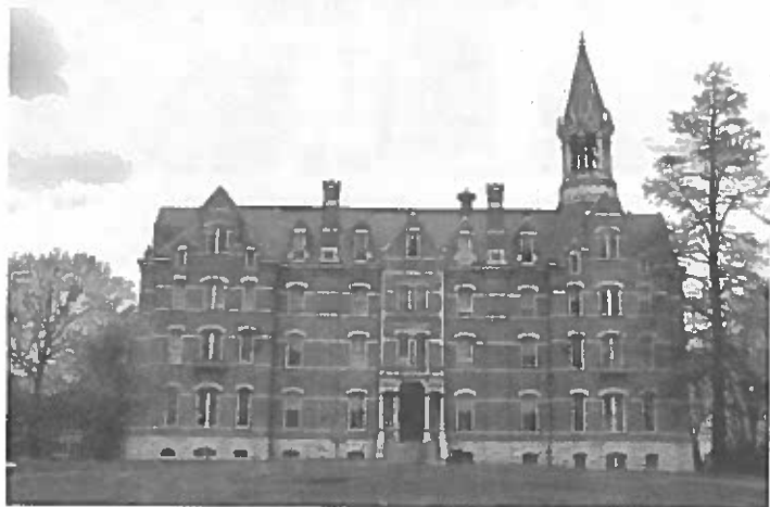
Jubilee Hall was constructed in 1876, and was one of the first brick buildings on the Fisk University campus. This National Historic Landmark was named in honor of the Fisk Jubilee Singers. Photo by Jeanne Cyriaque
