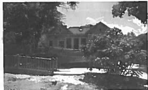
An ADA-accessible ramp was added to the rear entrance of the Alma Thomas childhood home.
