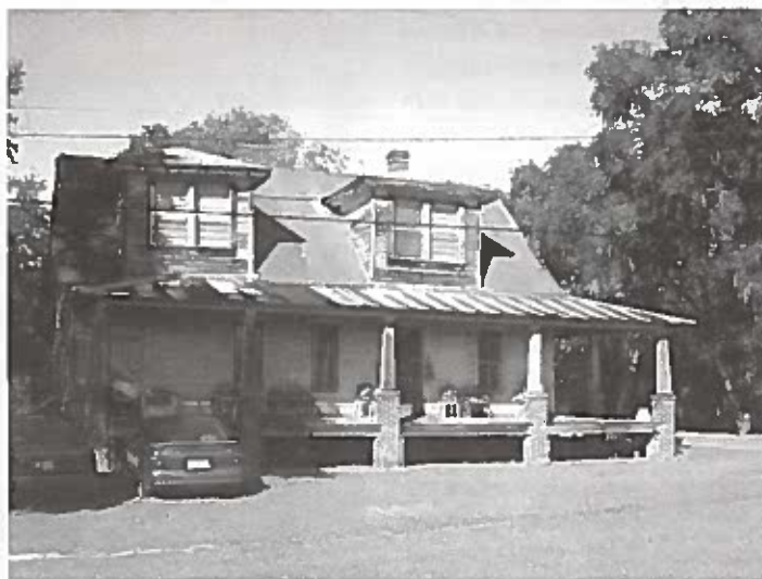
This circa 1840s residence was spared in the burning of Darien in 1863. For many years, it was the residence of Professor James Grant, an African American educator. Naomi Cooper and Derek Henley, descendants of the Grant family, live in this historic house. The Grant House is a contributing resource in the Vernon Square - Columbus Square Historic District, listed in the National Register of Historic Places on March 14, 1985. Photo by Jeanne Cyriaque
