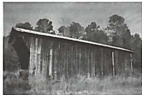
This section of the bridge that once spanned Wehadkee Creek in Troup County is preserved by stewards of the Ida Cason Callaway Foundation.
