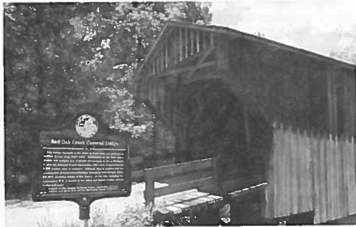
The Red Oak Creek Covered Bridge was built by Horace King circa 1840. It is the oldest covered bridge in Georgia, and was listed in the National Register of Historic Places on May 7, 1973. The bridge truss is constructed from heart of pine boards, and over 2,500 treenails, each approximately a foot long, hold it together. Photo by Jeanne Cyriaque
