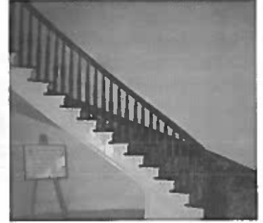
Horace King is credited with rebuilding this spiral staircase in the restored Alabama State Capitol.
