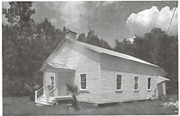
New Ogeechee Missionary Baptist Church was listed in the National Register of Historic Places on August 8, 2001. Photo by James R. Lockhart
