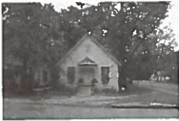
The Clay Street YMCA building is a community landmark building in Thomasville's Stevens Street Historic District. It was built circa 1890 to provide recreation services to the African American community. Today, the building functions as True Vine Church of Deliverance. It is owned by the Douglass High School Alumni Association. Photo by Jeanne Cyriaque
