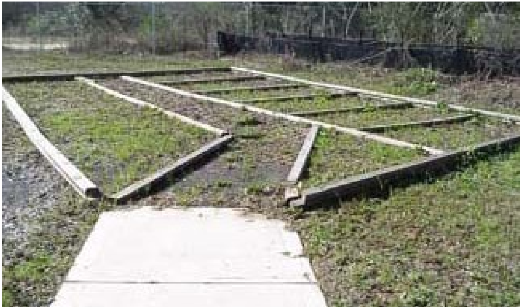
Not Acceptable No fence; overgrown with weeds.
