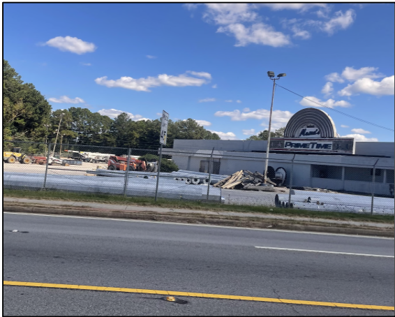
Site facing north along Covington Highway
