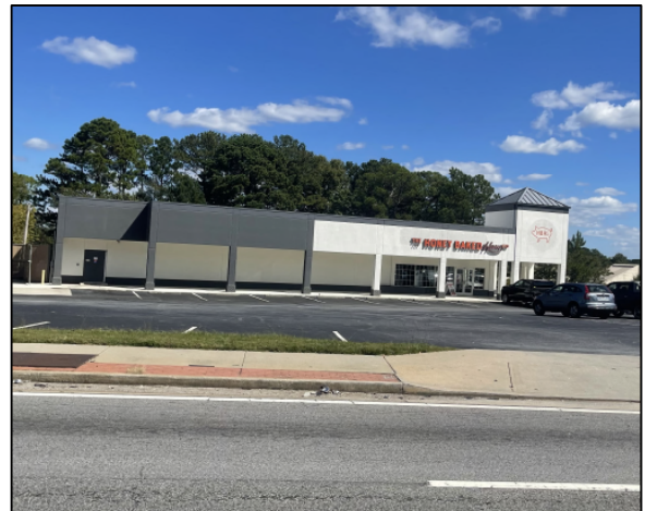
Honey Baked Ham to the west of the site along Covington Highway
