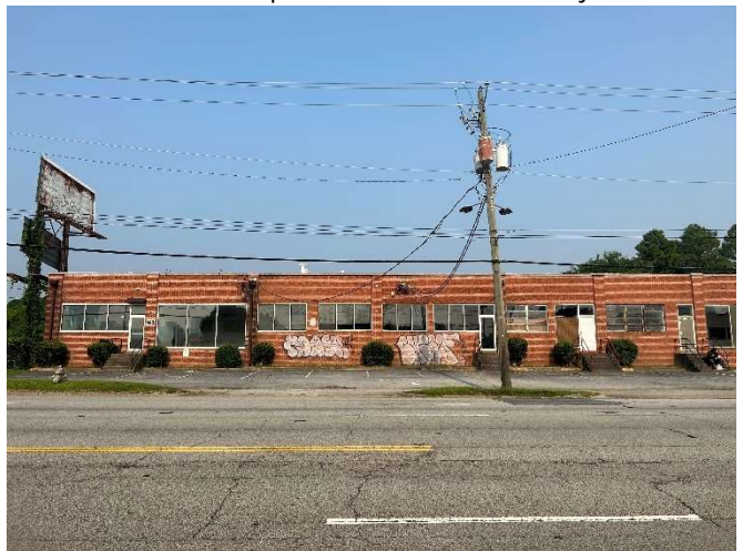
Vacant offices west of Subject site
