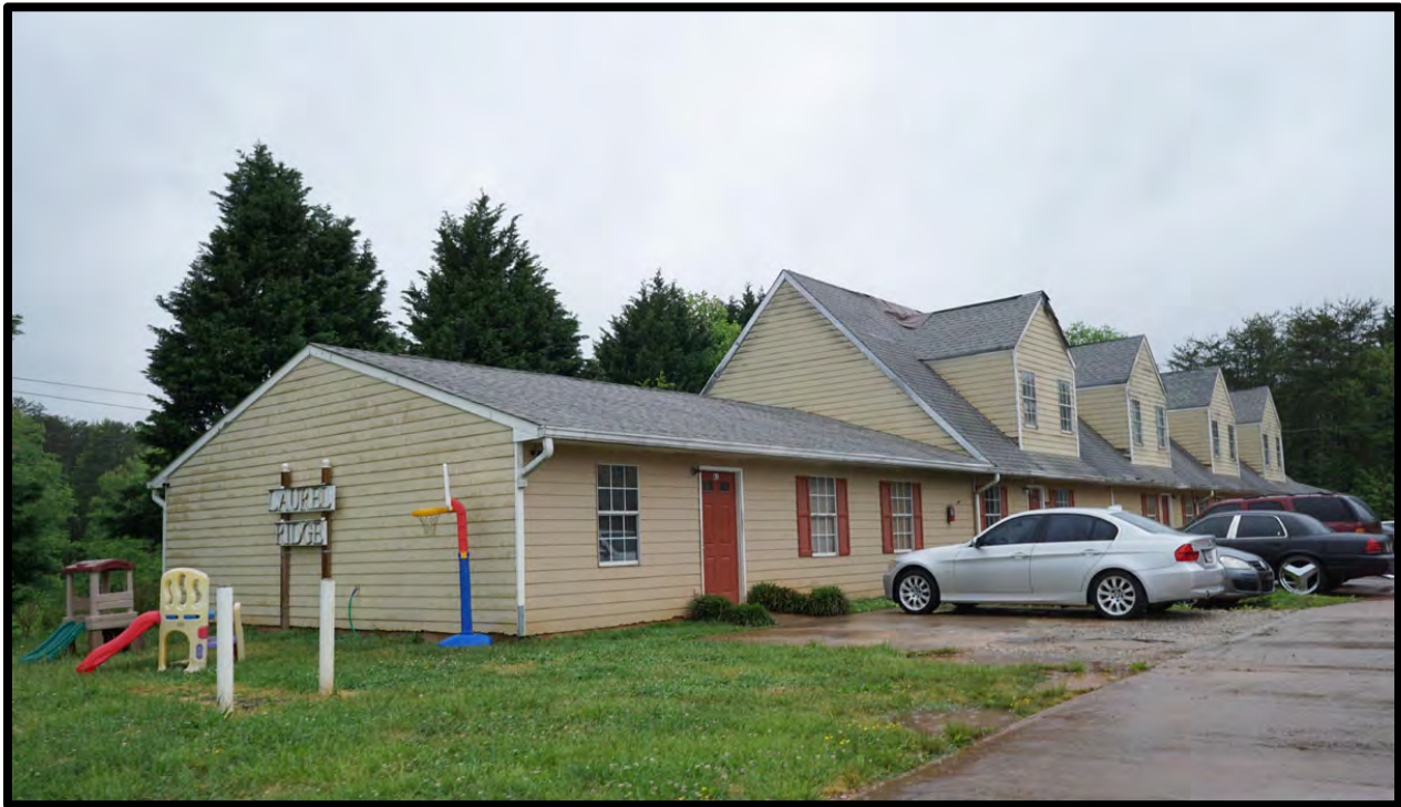
Photo 12 Laurel Ridge Apartments (adjacent to the site to the south)
