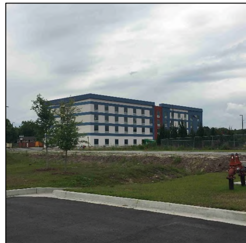
Home2 Suites hotel under construction
