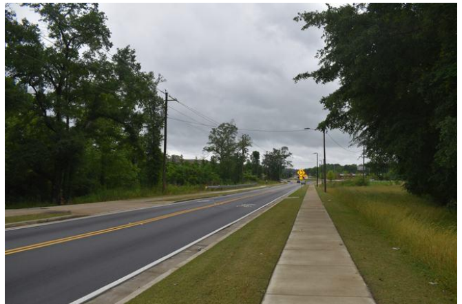
View south of the Subject site on Brennan Road
