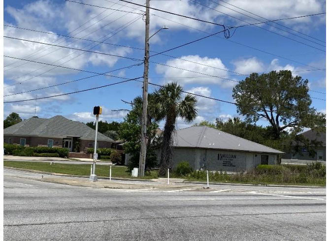
Commercial uses north of the Subject site on Glynn Avenue
