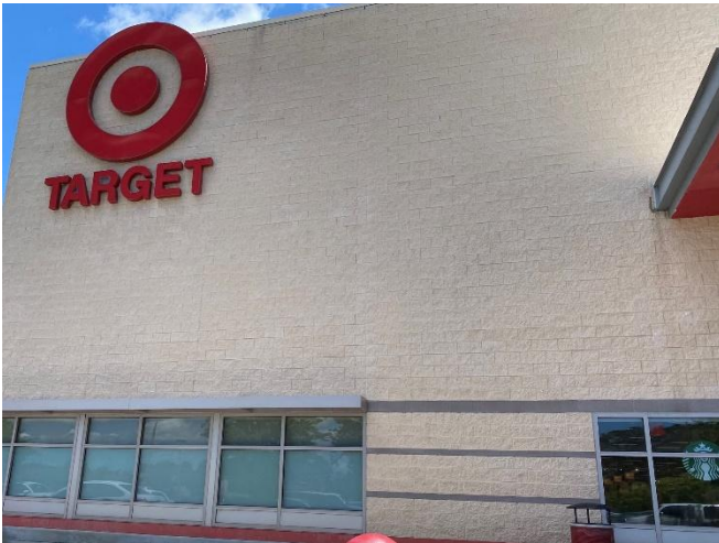
Shopping center northwest of the Subject site
