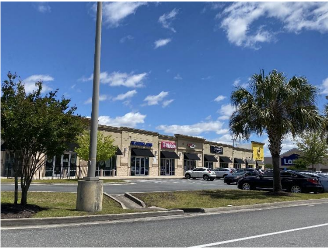
Shopping center northwest of the Subject site
