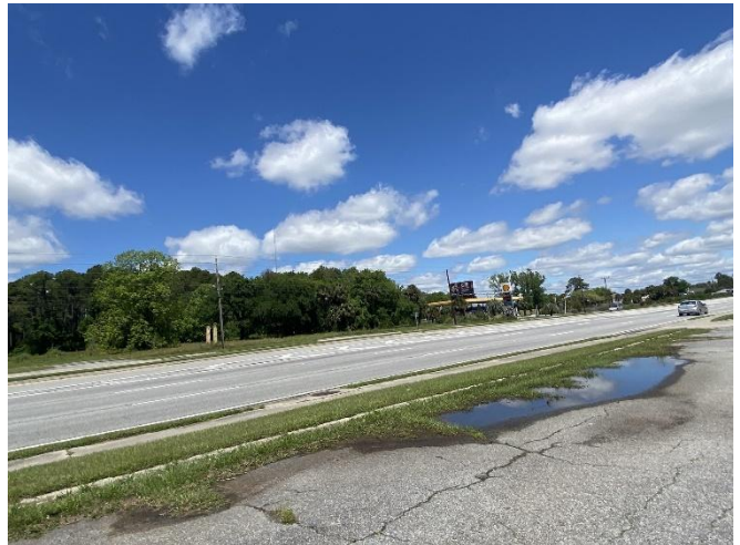
View north on Glynn Avenue
