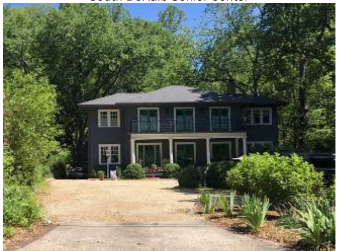
Typical single-family homes in the Subject's neighborhood
