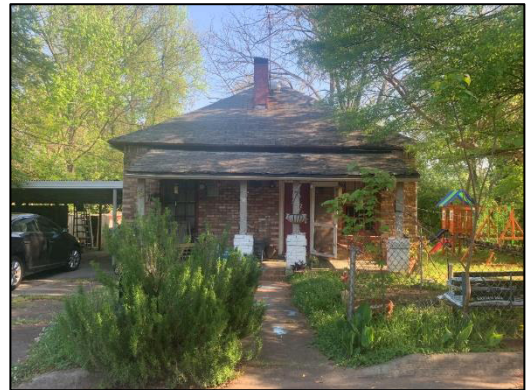
Single family dwelling to the south on Burnap Street
