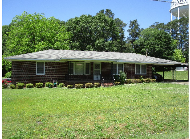
Single-family home in Subject's neighborhood
