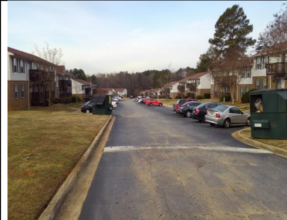
Subject Parking Lot
