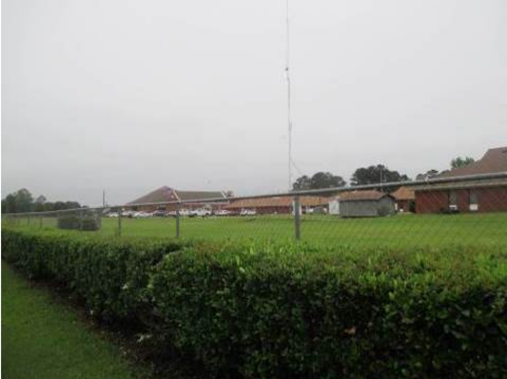
View to the North
