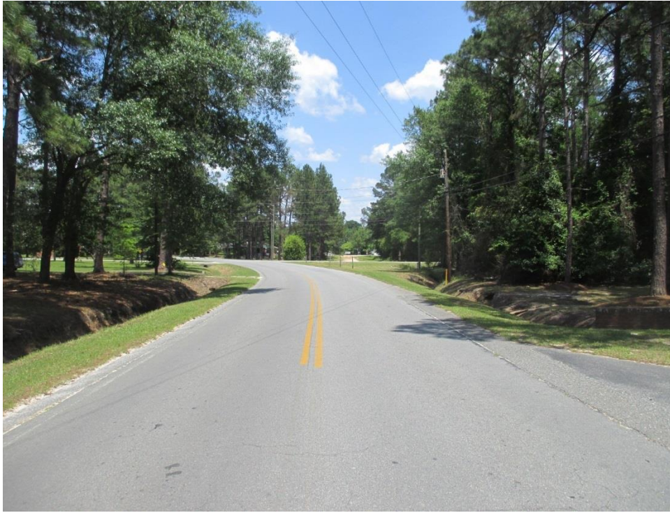
View to the North
