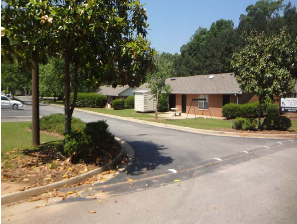
View to the North
