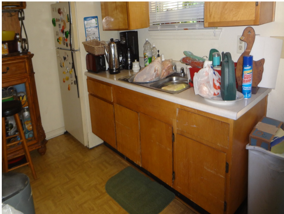
View of Kitchen – One-Bedroom Unit
