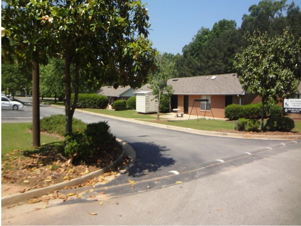
View to the North
