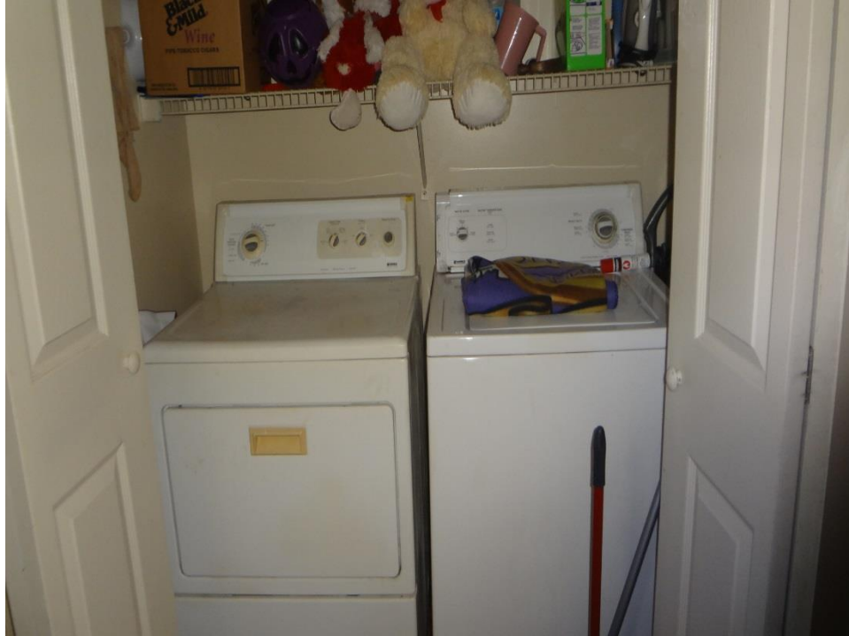
View of Utility Area – Two-Bedroom Unit
