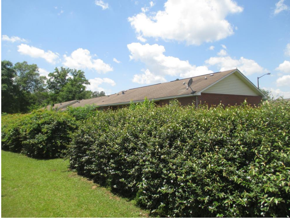
View to the North
