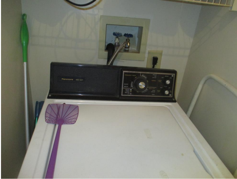
View of Utility Area – One-Bedroom Unit
