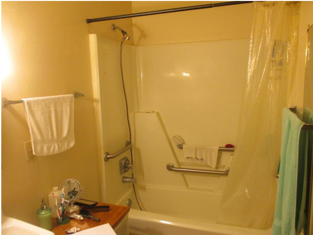
View of Bath – One-Bedroom Unit
