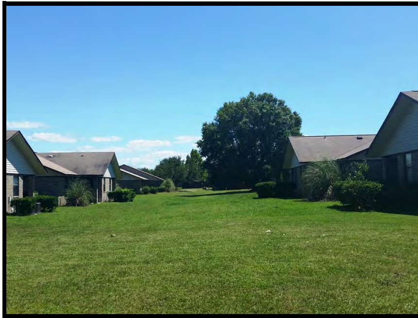
View of site from the north
