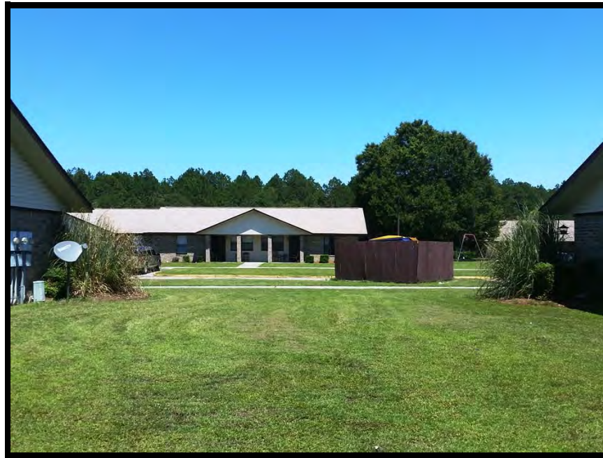
View of site from the west
