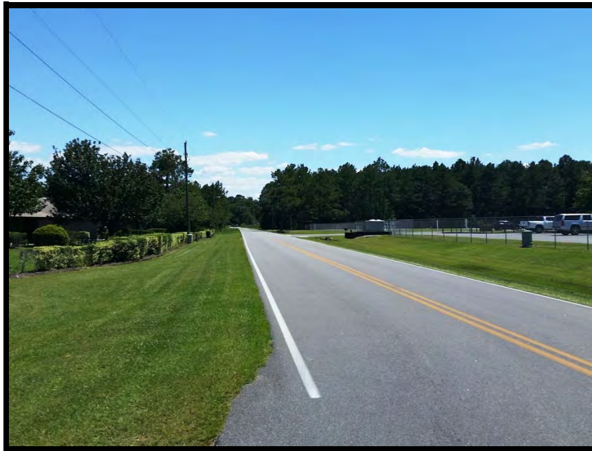
Streetscape- South View of Carswell Street
