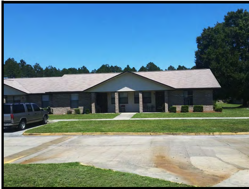
Typical Building Exterior
