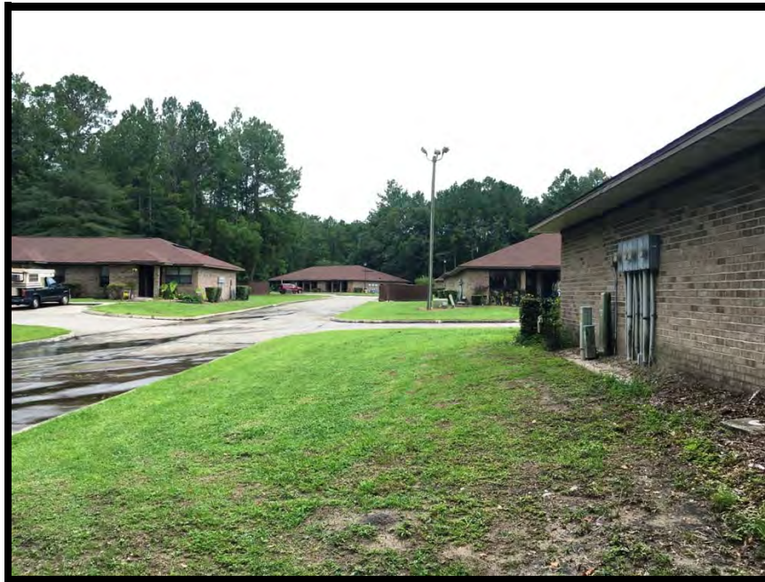
View of site from the north
