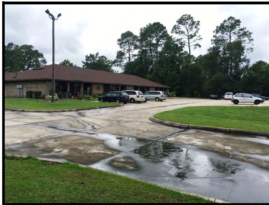
View of site from the northeast
