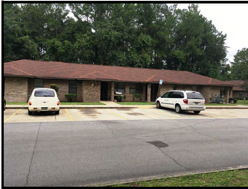
Typical Building Exterior
