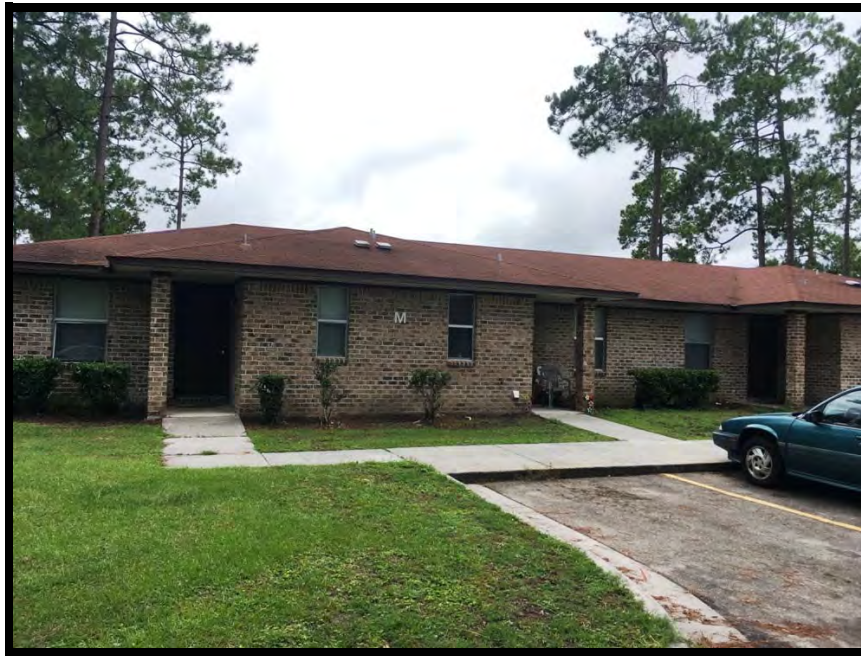
Typical Building Exterior
