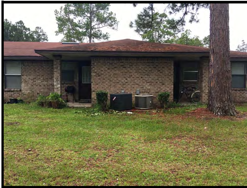
View of site from the north
