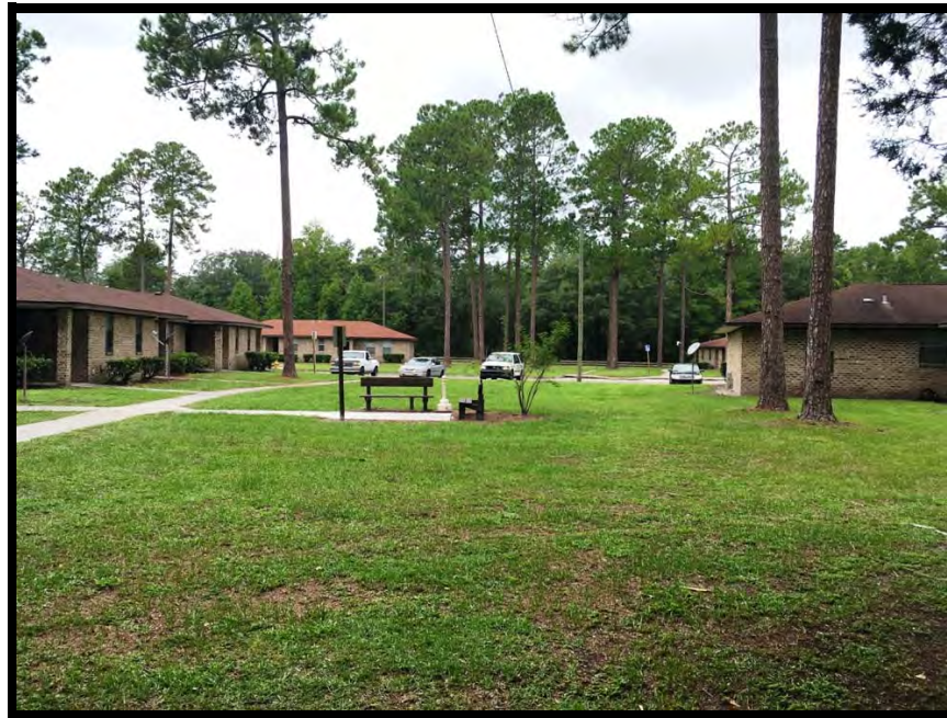
View of site from the east
