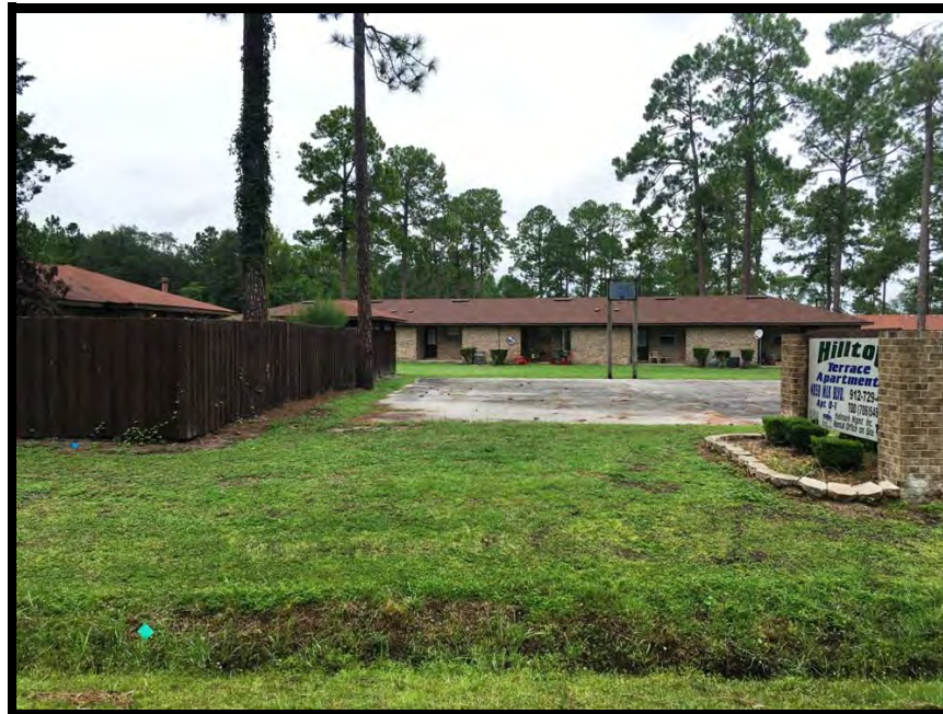
View of site from the south
