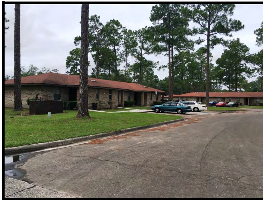
View of site from the southeast
