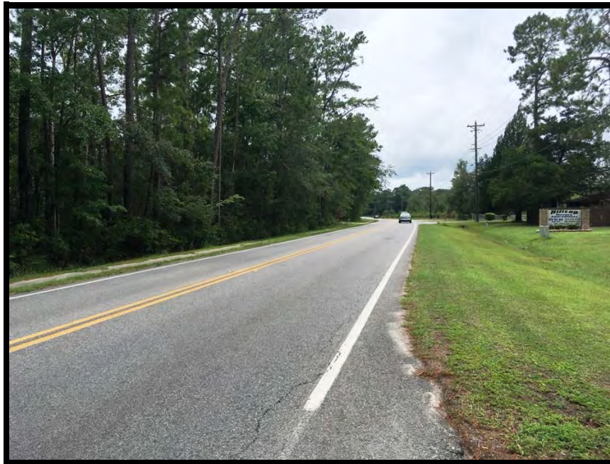
Streetscape: West view of Martin Luther King Boulevard
