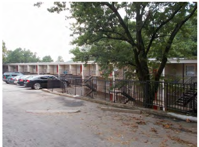
View of Rolling Bends Phase II to the south
