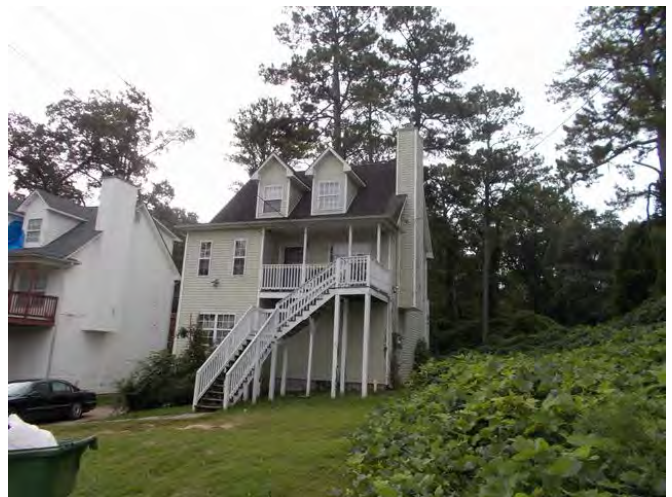
Typical single-family home in the Subject's neighborhood
