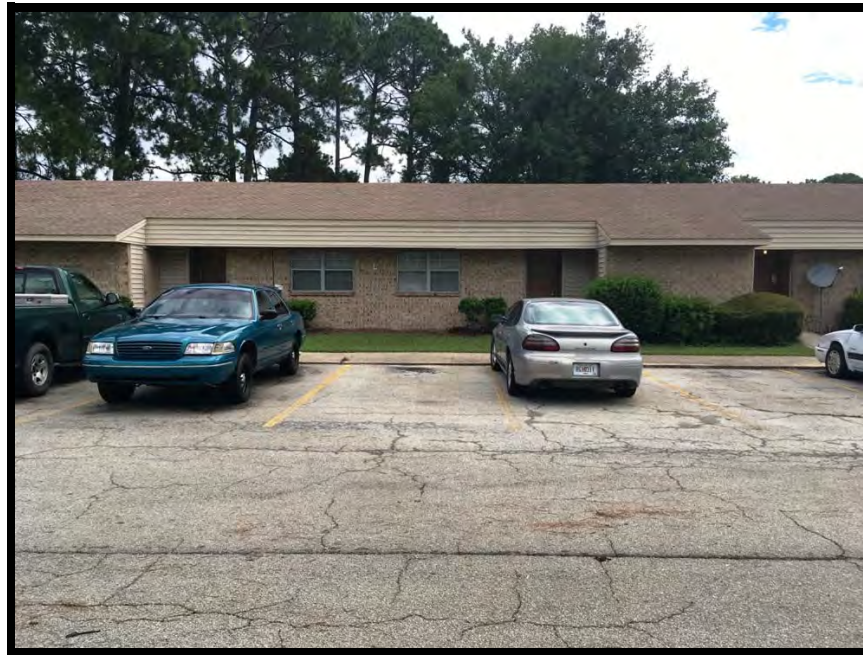
View of site from the southwest
