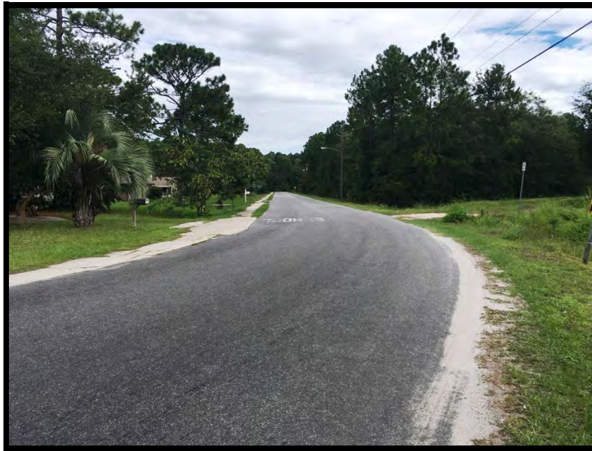
Streetscape: North view of Martha Street
