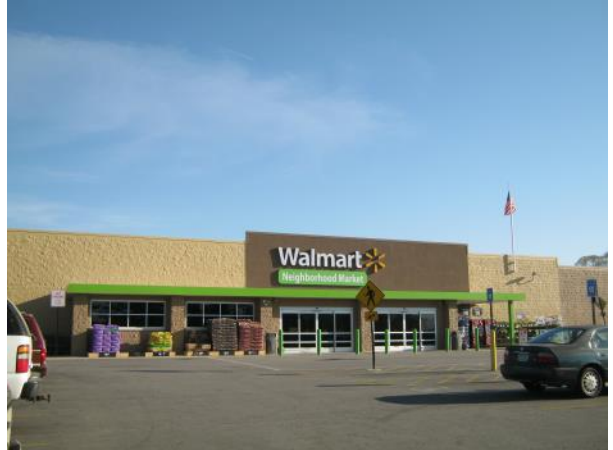
Typical retail uses along Lafayette Parkway
