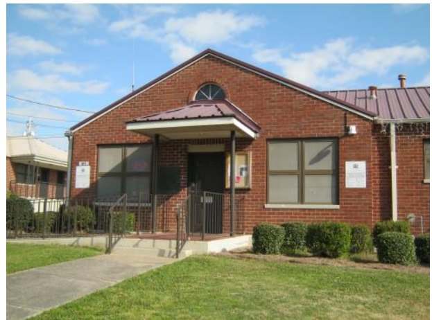
Management office exterior
