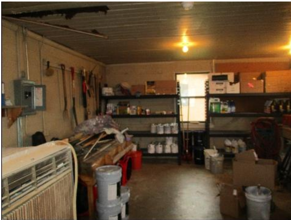
View of Maintenance Area
