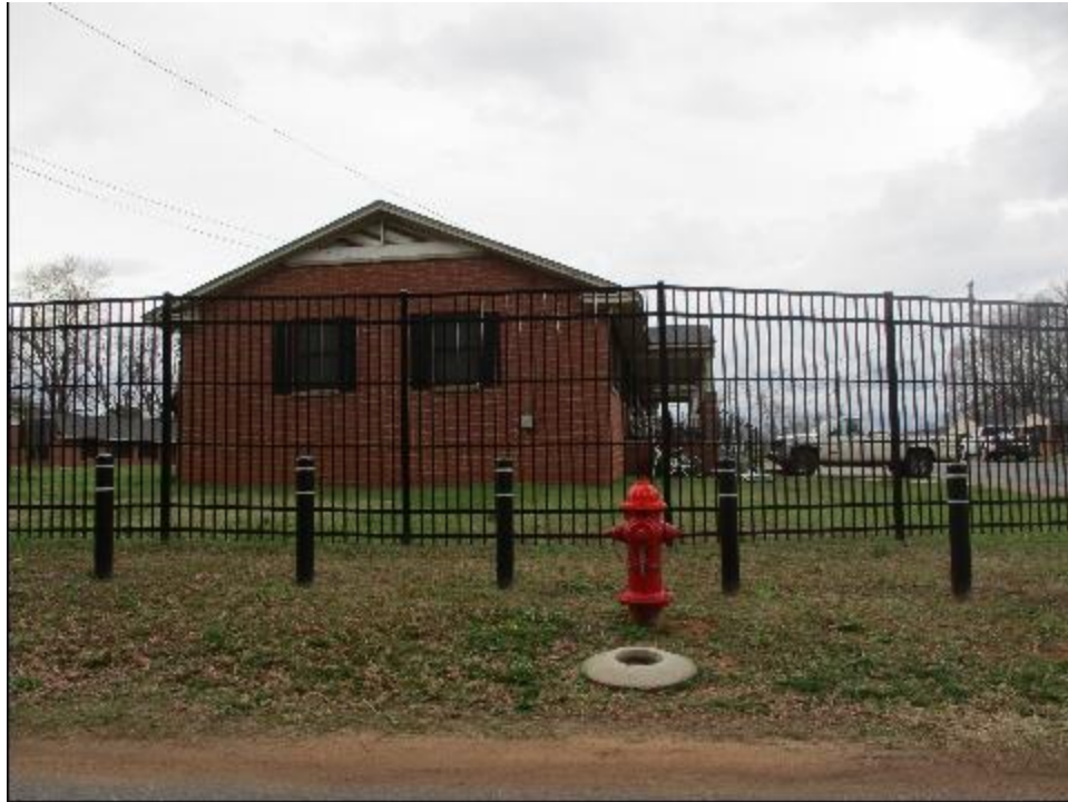
View of Perimeter Fencing
