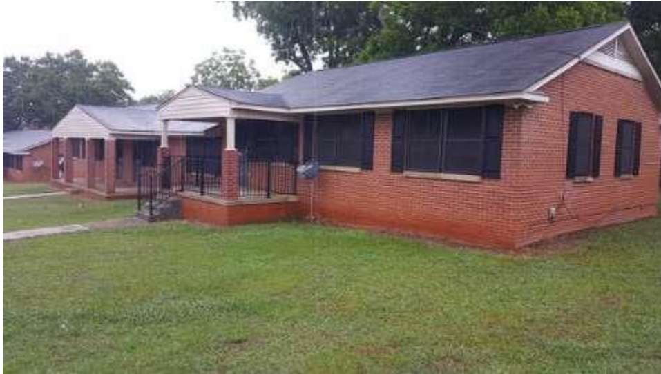
View of Exterior
