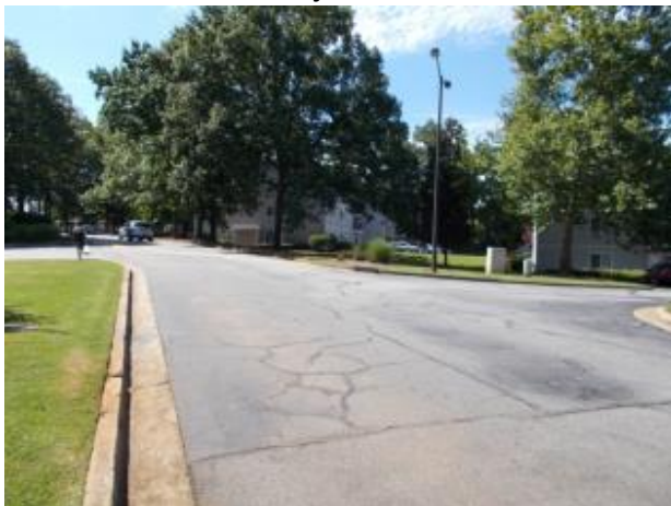
View south on Hillcroft Lane
