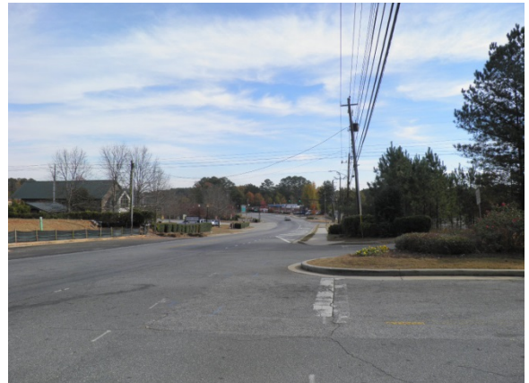
Looking easterly along Arnold Mill Road (Photo Taken on November 22, 2016)
