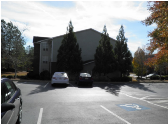
Exterior of an apartment building (Photo Taken on November 22, 2016)
