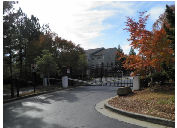
Gated entrance (Photo Taken on November 22, 2016)
