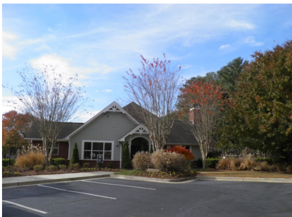
Leasing office/clubhouse (Photo Taken on November 22, 2016)
