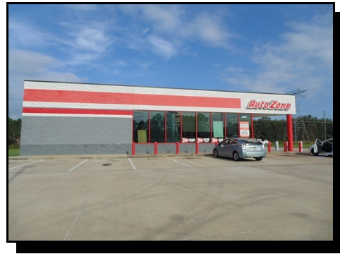
(8) Autozone, .1 mile from site.
