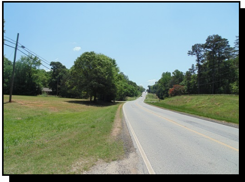
(3) Site to the left, north to south.
