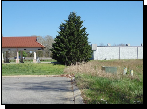
(3) Site entrance right, off service road, west to east.
