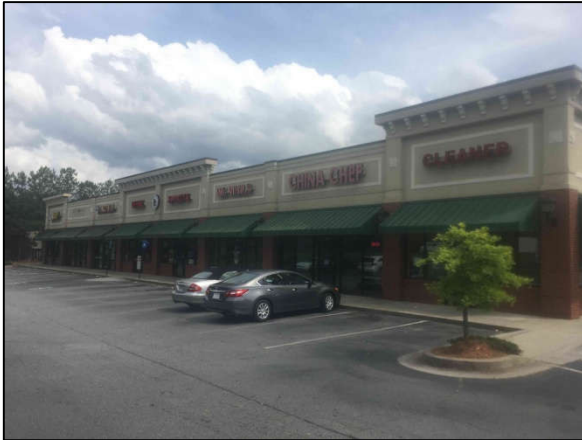
A retail strip center bordering the site to the south.
