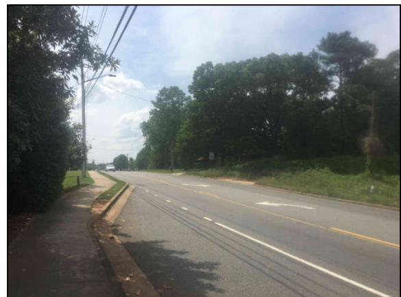
Baker Road facing west, site on right.
