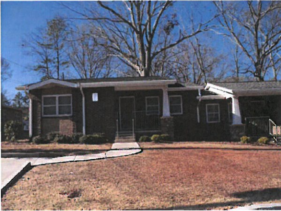
Unit Exteriors - Remodeled
