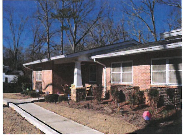
Unit Exteriors - Remodeled
