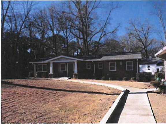
Unit Exteriors - Remodeled
