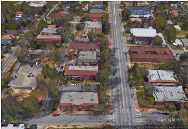
Aerial of Six Buildings, Looking From South To North
