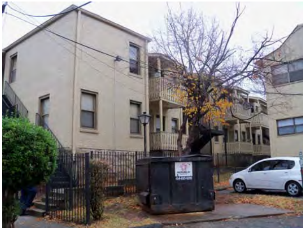
West Side of Subject Block Along Latta Street
