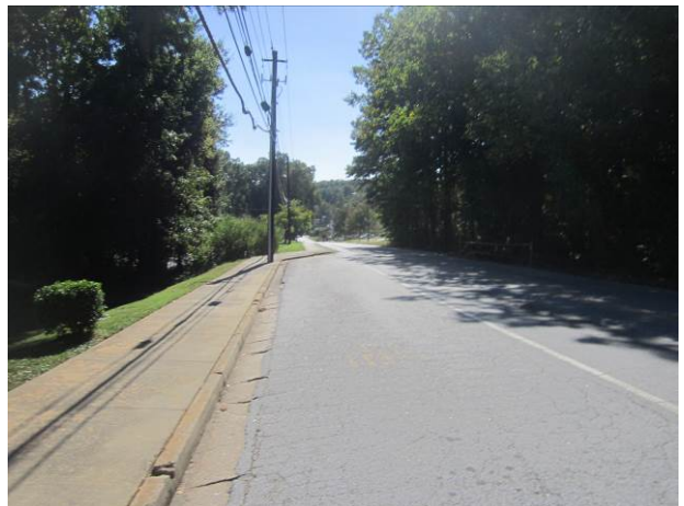
View along Whites Mill Road facing southwest
