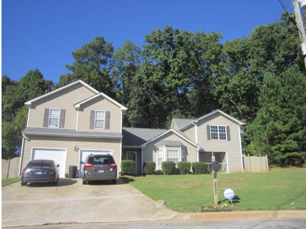
Single-family home to the south of the Subject site (facing the Subject site)
