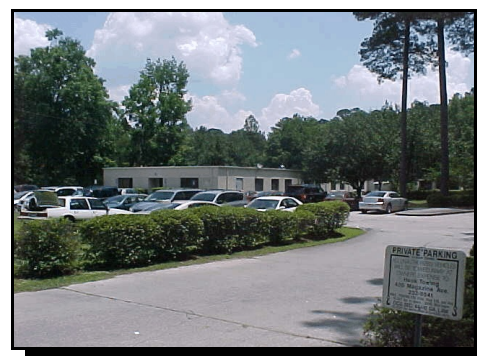
(4) Place @ Pooler nursing home east of site, off Rogers St
