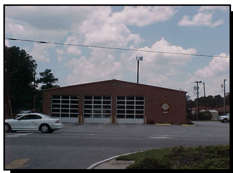
(6) Pooler fire station, .3 miles north of site.
